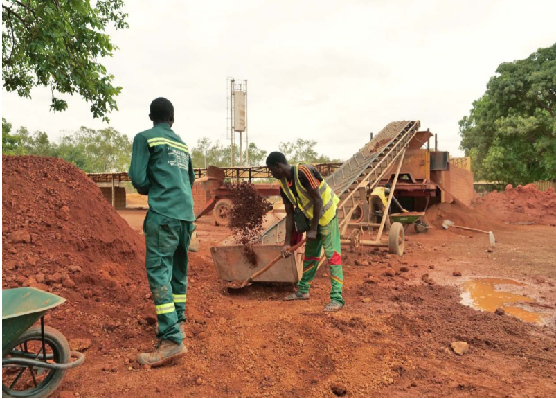
ZI Matériaux workers on site
