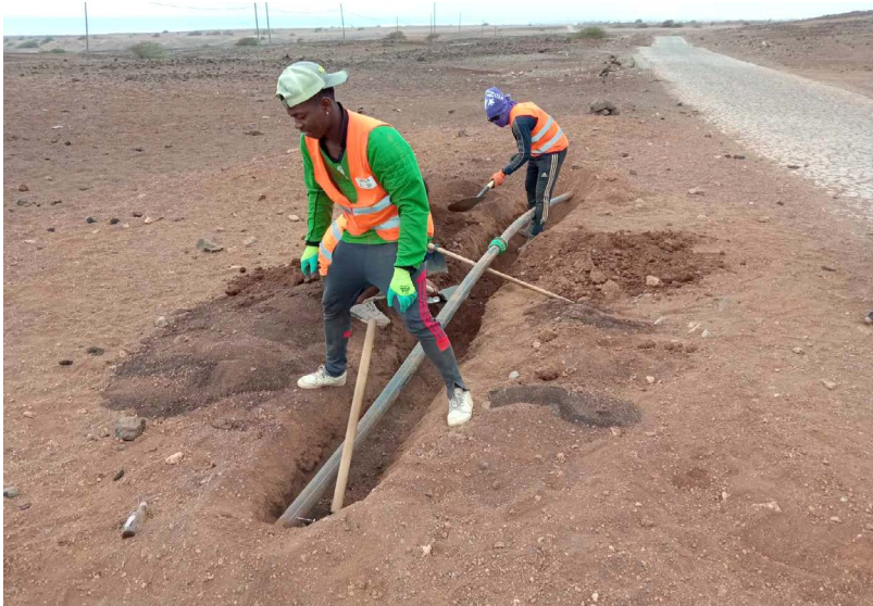
Works to optimise Maio’s drinking water network
